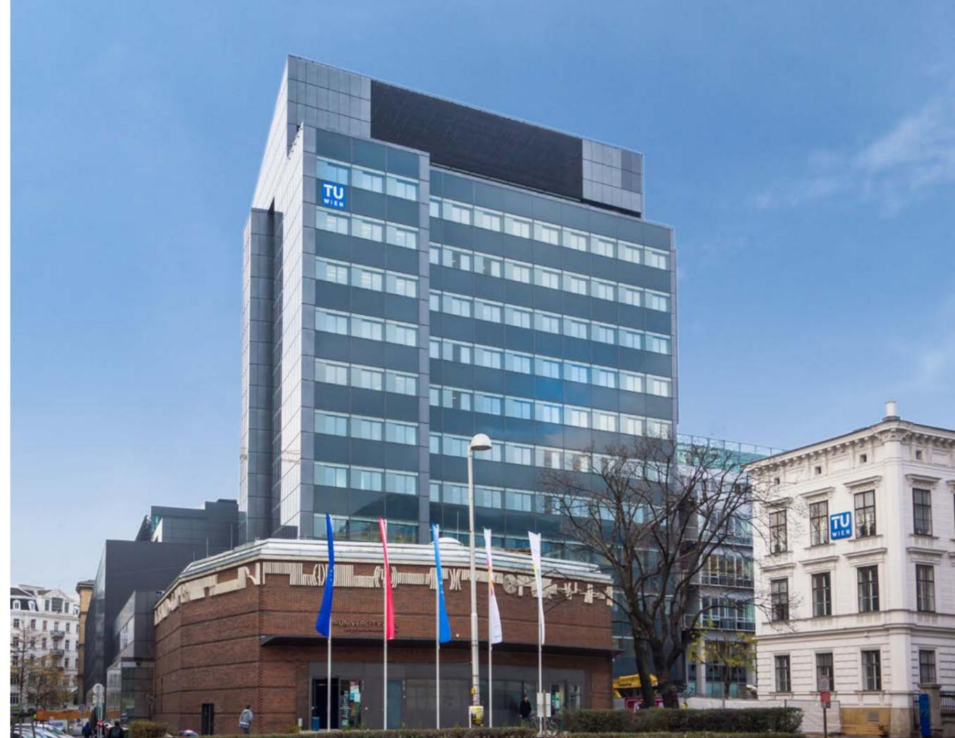
The former Chemistry block of the Vienna University of Technology, with a net floor space of 13,500 square metres on eleven floors, was converted into Austria’s largest plus-energy office building in the course of a general renovation and at the same time became a showcase building unique throughout the world. It’s remarkable that the plus-energy standard was achieved here with an existing high-rise building from the 1970s – with primary energy, on site.
